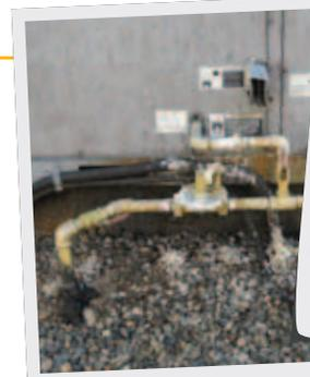
Bird Droppings Corrode Pipes
