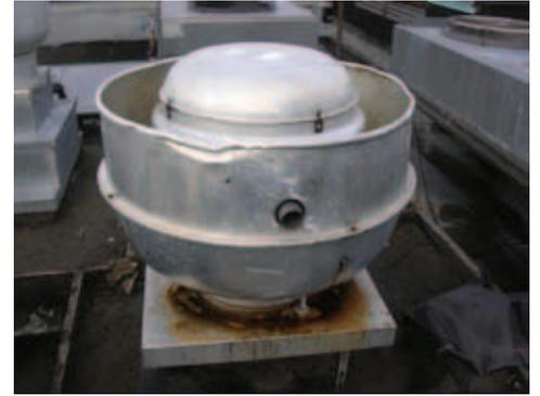
*Older Equipment Leaking onto Roof*
